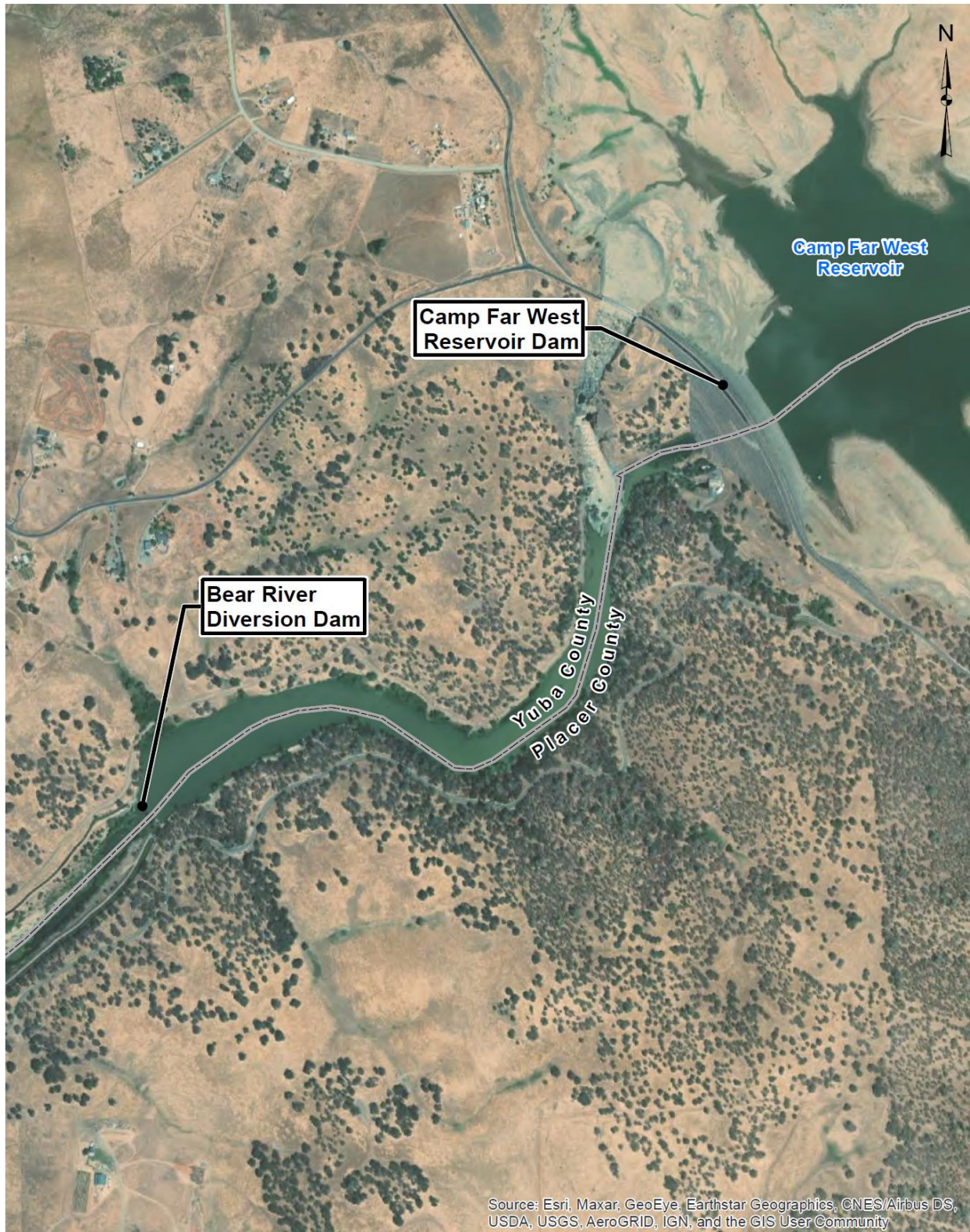
Figure I-2 SSWD – Facilities in Yuba County
